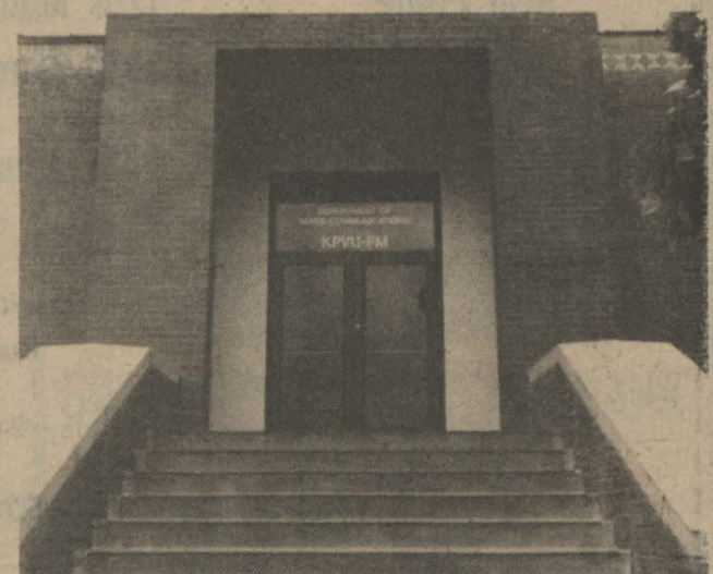
RADIO STUDIOS and business offices are being completed in Communications Center.
