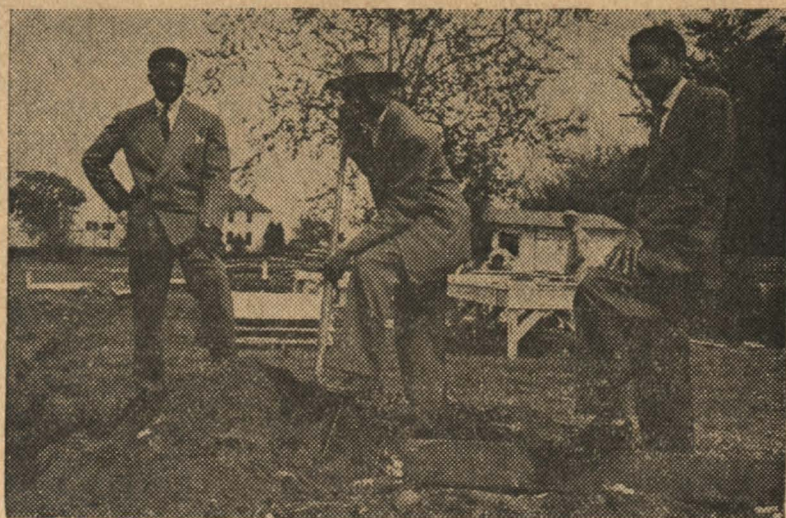
GROUNDBREAKING FOR NEW ENGINEERING BUILDING
