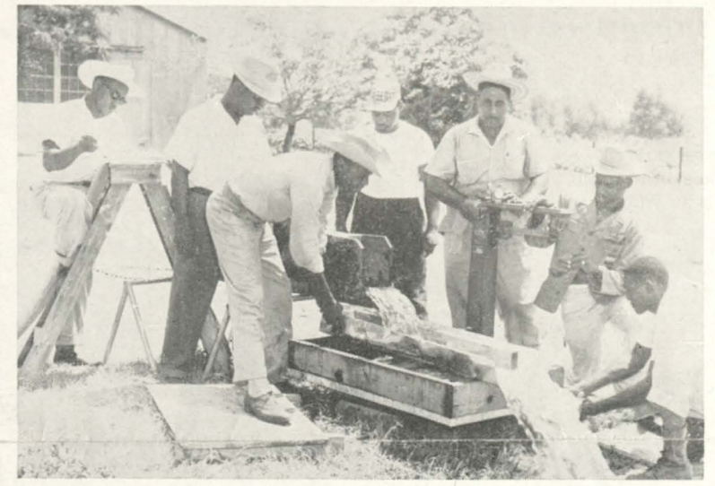
FARM DRAINAGE — A graduate class in farm drainage is shown calibrating a modified 3-inch Parshall flume which was built as a class project during the summer session. W. O. Mack Agricultural Engineer, was in charge of the experiment which provides a very accurate method of measuring water flowing in an open ditch and which has a very practical application in open channel supply for irrigation.
