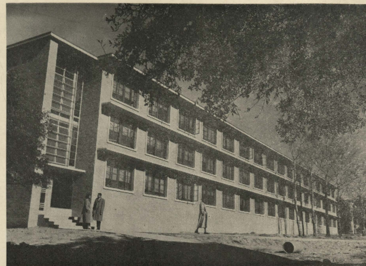
SUAREZ HALL . . . first picture of the recently occupied dormitory for women. The $350,000 structure is modern and first-class in every detail. It houses 247 senior co-eds, with excellent facilities for recreation and social entertainment. It is named for the late Miss Mary Suarez, Dean of women at the college for many years, and idolized by thousands of young women who have called Prairie View their home.
