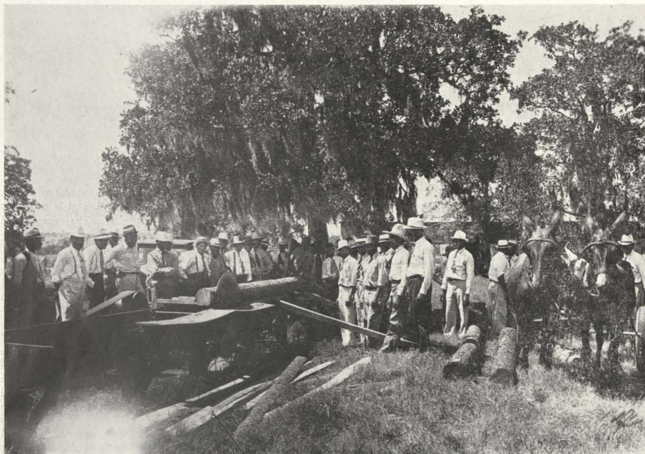
Cooperative Saw Mill owned by farmers of Fayette County sawing lumber at the 31st. Annual Farmers Short Course at Prairie View, Texas. With the aid of this saw mill a community house, with offices for a Farm and Home agent, has been built at LaGrange, Texas, with the assistance of the Negro Agricultural Agent.
