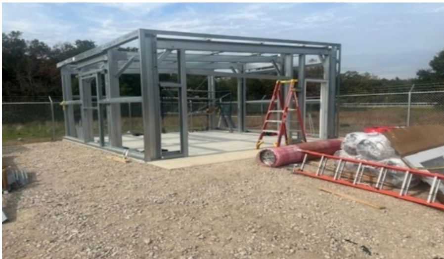
Fig. 96 PV Platform under construction [179].
