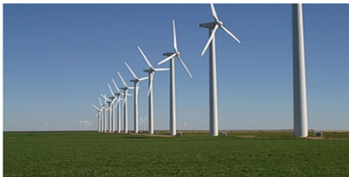
Fig. 9 Brazos Wind Turbine Towers [27]
