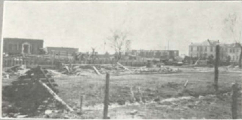
Mechanical Storeroom Boys' Dormitory Construction Work
