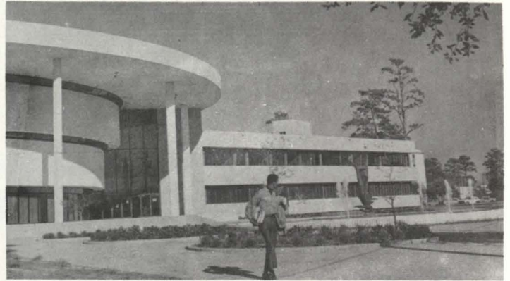
Martin Luther King Bldg.
