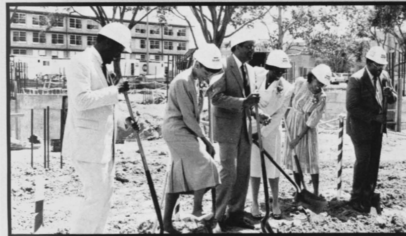
President Pierre and McKee Contractors at the Ground Breaking Ceremony.
