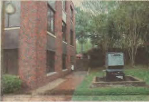
A.I. Thomas' new electrical generator.
